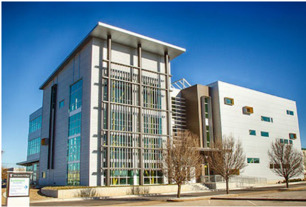
TJC West Campus Energy Center (Credit: John Jackson at Holland Engineering)
